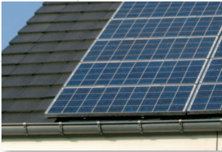
Afb. 1 Montage bovenop de dakbedekking.
